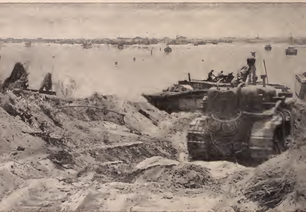
BULLDOZERS CLEARED ROADS to beach dumps for the tracked amphibious vehicles which carried the supplies from the reef to storage and dispersal areas on shore. Along the reef (at center) a crane loads a tractor; the transport ships are anchored farther out to sea.
